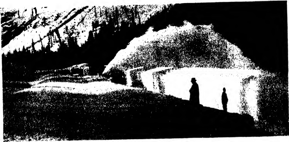
CUTTING A ROADWAY THROUGH STEVENS PASS IN WASHINGTON STATE AT THE END OF A WINTER SEASON.
